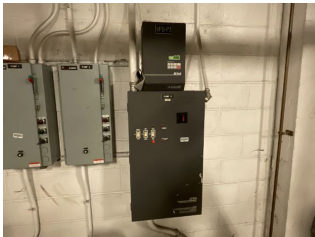
Variable Frequency Drive - 20 HP -1
