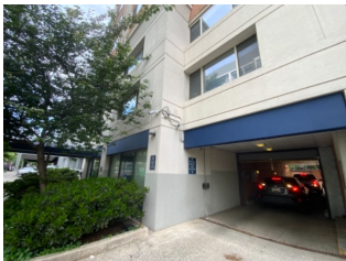
Exterior Limestone Wall Finish
