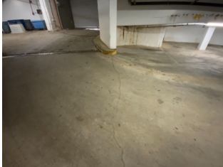
Service Parking Lot - Concrete Concrete Parking Lot
