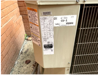
Air-Cooled Heat Pump - 3 Ton
