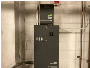
Variable Frequency Drive - 20 HP -2
