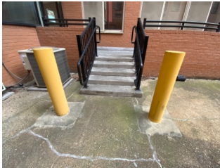
Exterior Stairs - Concrete - Medium Exterior Stair
