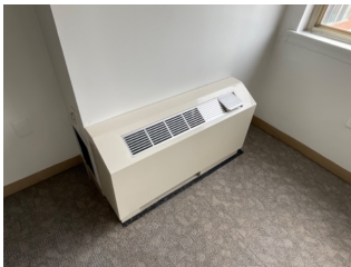
Heat Pump - Water Source
