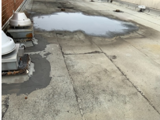
Modified Bitumen Modified Bitumen Roof
