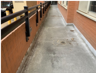
Exterior Ramp - Accessible - Concrete Ramp
