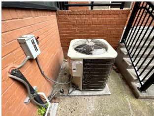
Air-Cooled Heat Pump - 3 Ton
