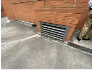
Metal Wall Louvers Metal Cover
