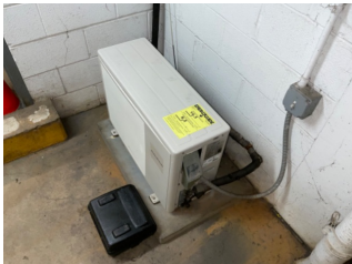
Split System Heat Pump - 3/4 Ton
