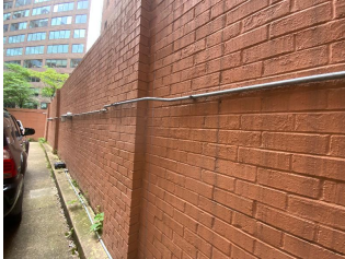
Brick Exterior Fence
