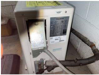
Split System Heat Pump - 3/4 Ton
