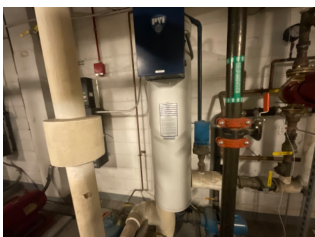
Water Heater -Instantaneous Electric *
